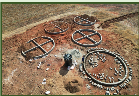
Construction of the bases for five water tanks.
